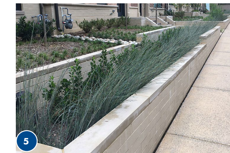
5 STORM WATER BOXES
